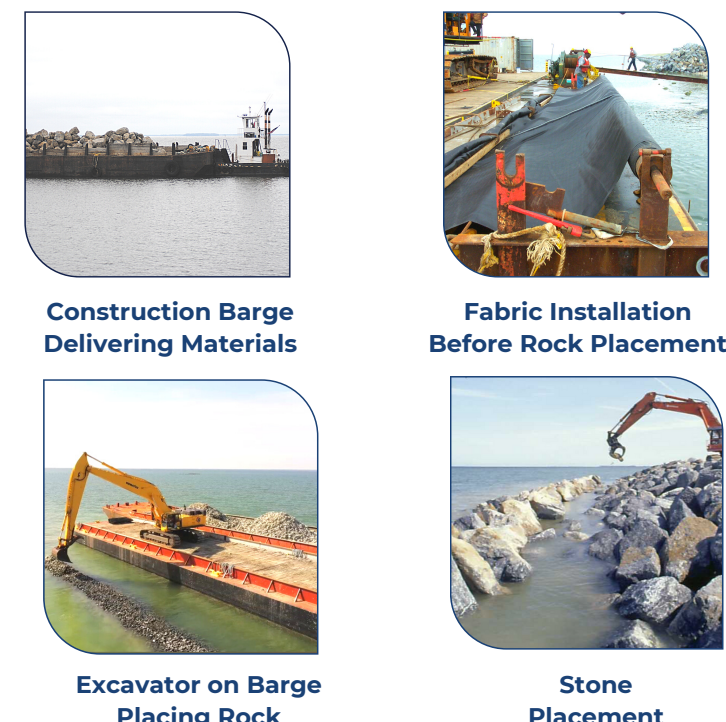
Figure 3. Examples of Equipment Used During Barren Island Phase I Construction
