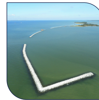
Construction of Southern Breakwater
